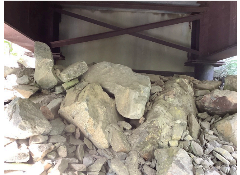
Right Bank Abutment when facing downstream
