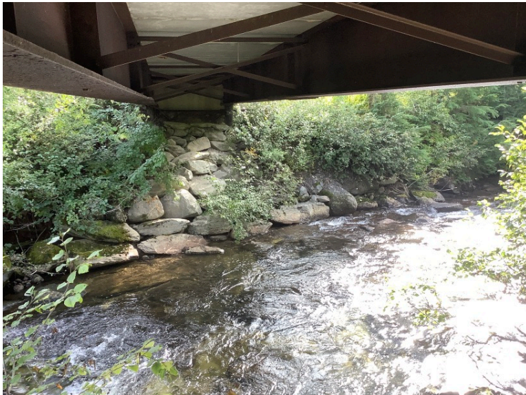
Left Bank Abutment when facing downstream
